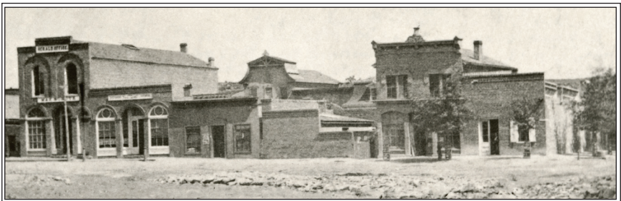
East side of Main Street looking north. The building on the left of the photograph housed the Herald, Silver City's only newspaper at the time. (1878) Courtesy of Silver City Museum
